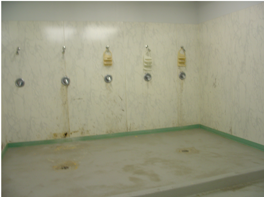
deteriorated wall finish in male showers
