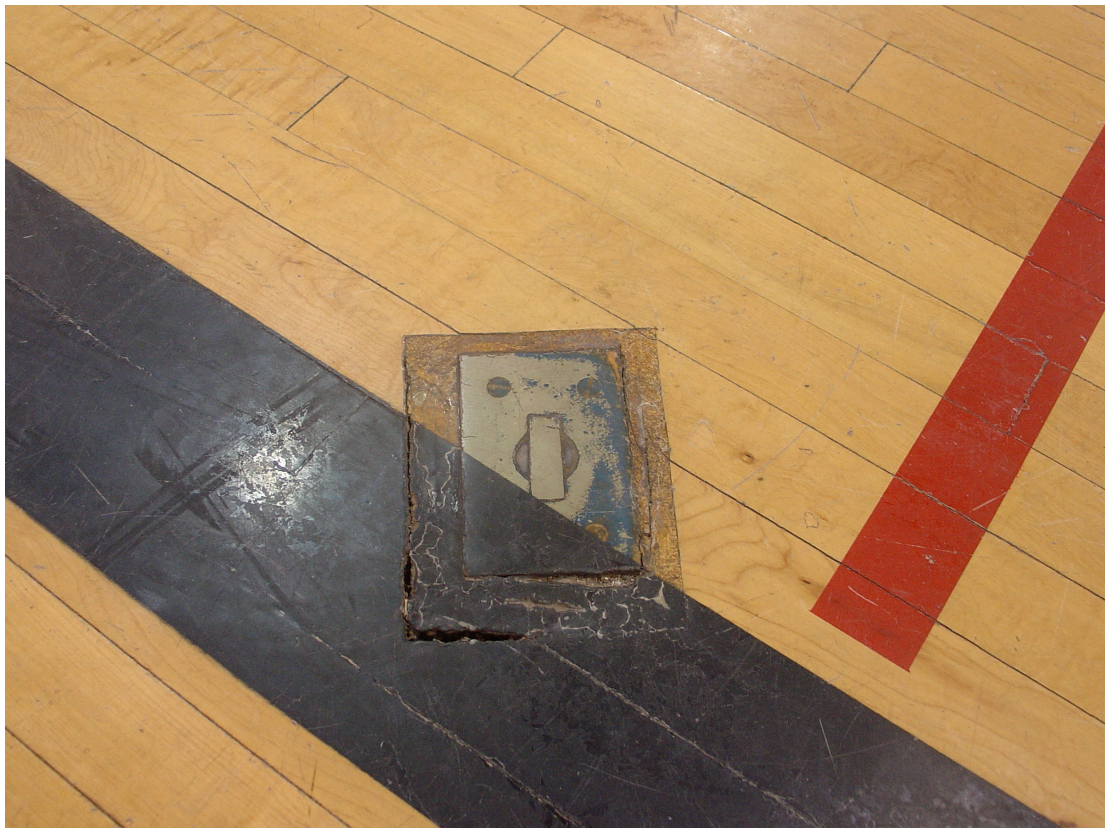
poorly installed gym floor insert
