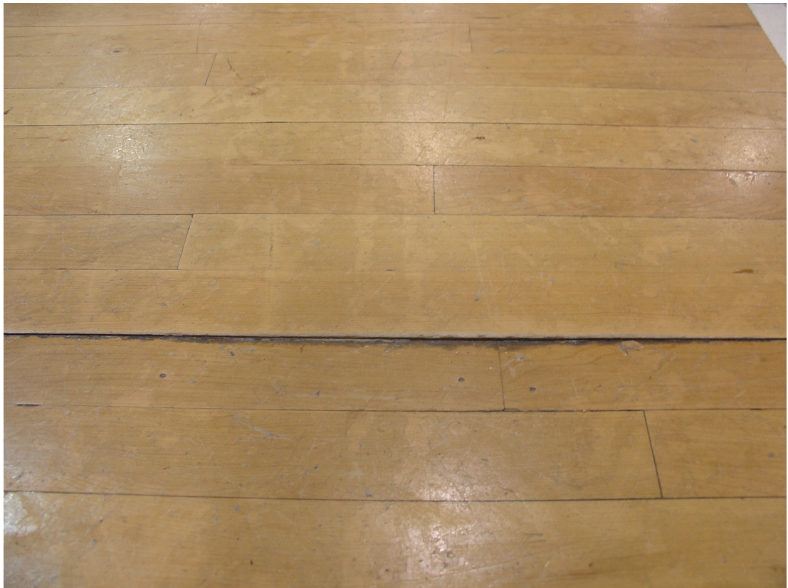
gymnasium floor plank deterioration causing ponding
