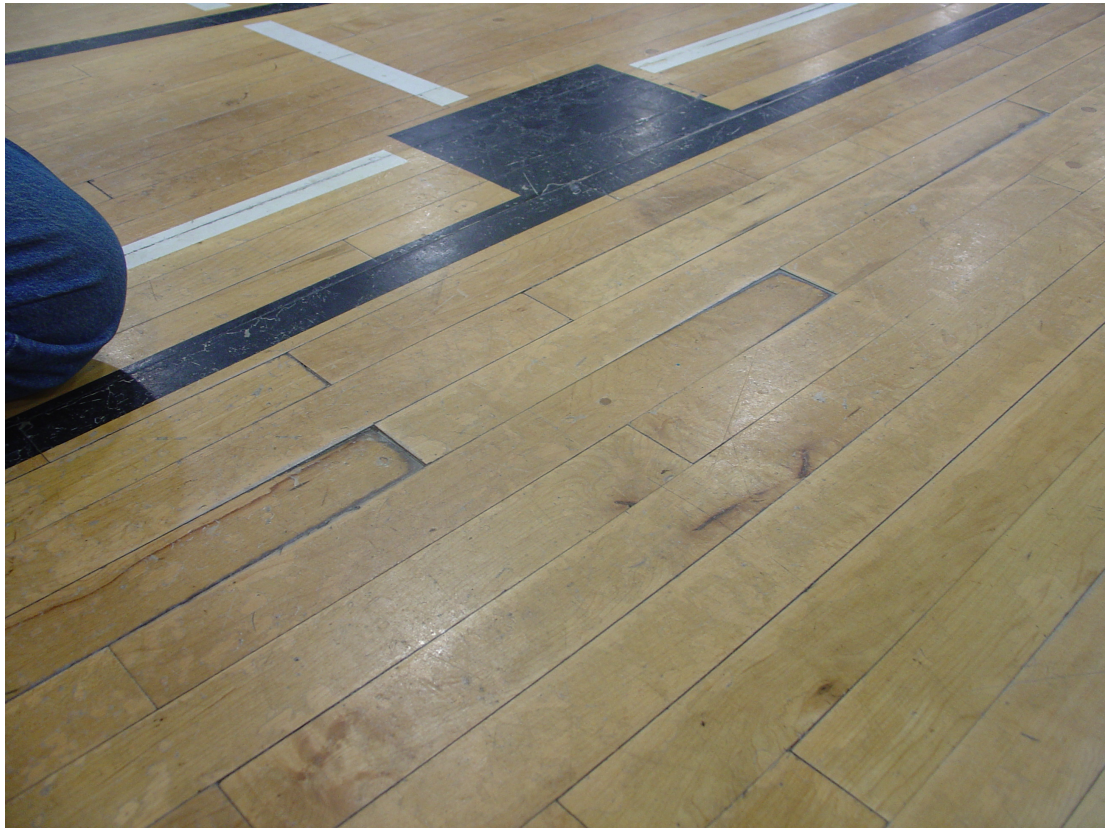
gymnasium floor plank deterioration causing ponding
