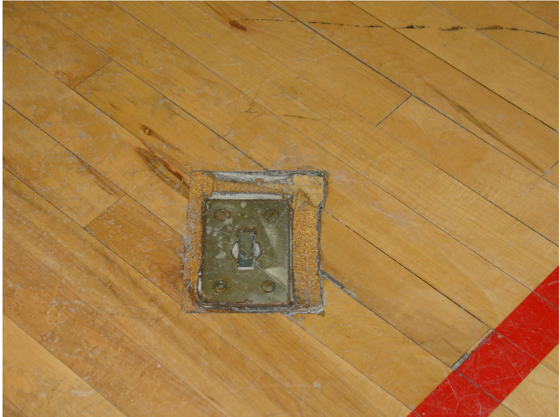
poorly installed gym floor insert
