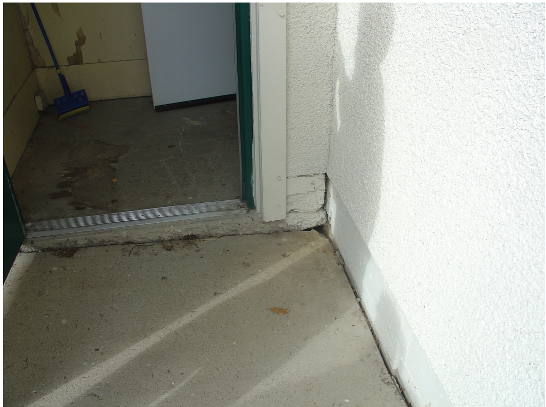
concrete pad settlement
