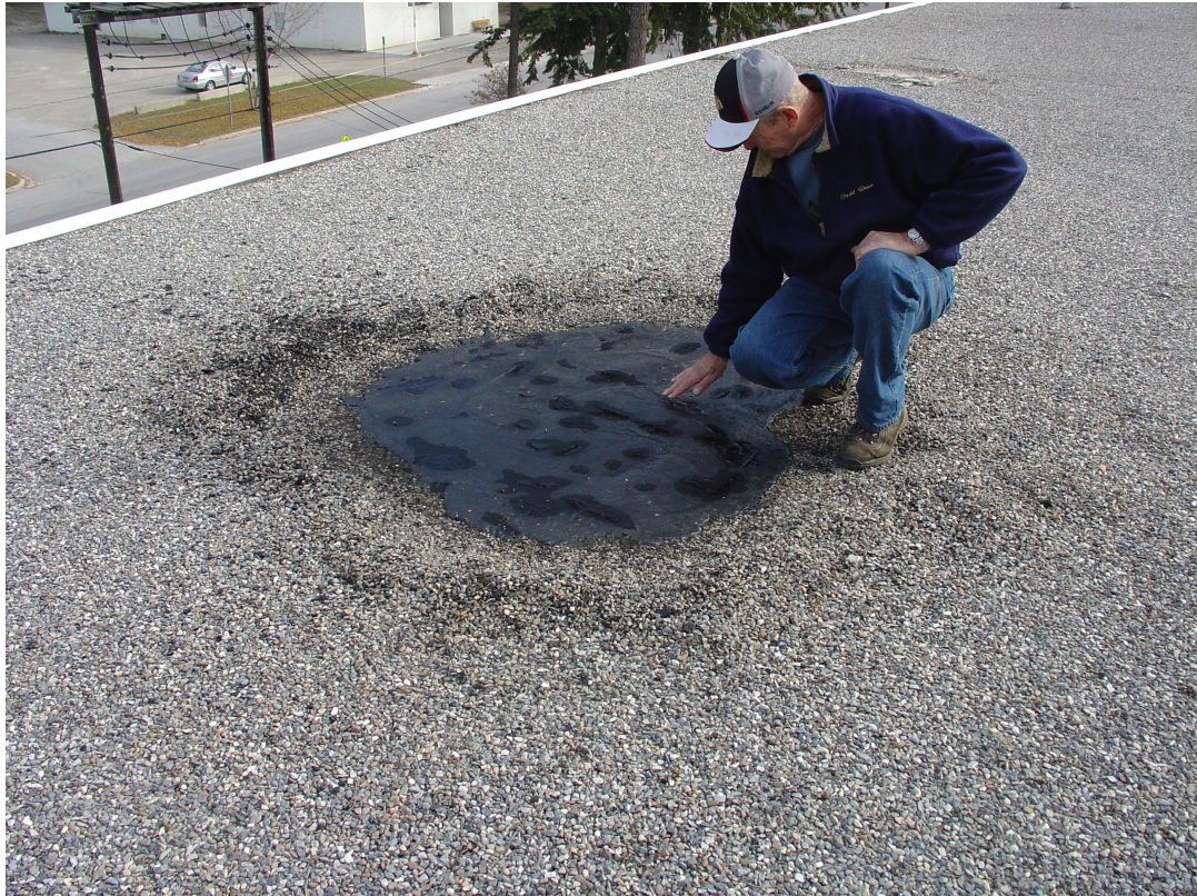
roof membrane blisters on the gymnasium roof
