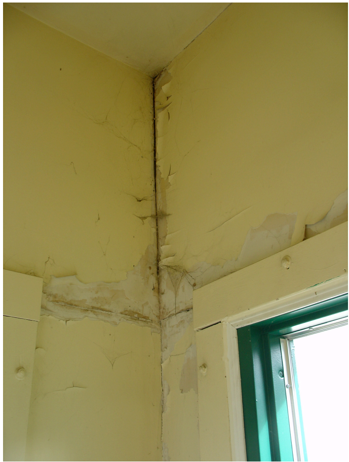
stucco wall interior damage
