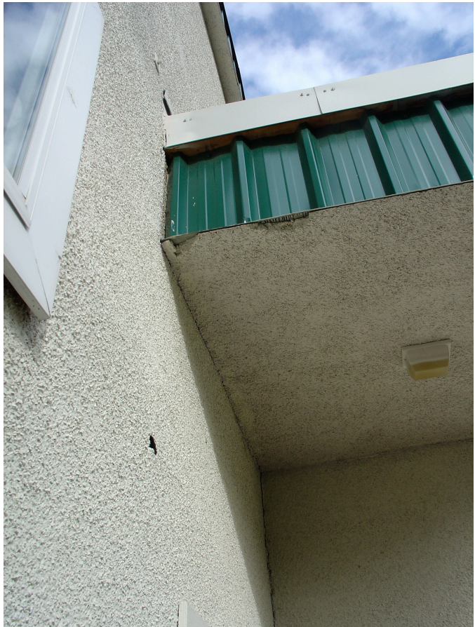
deteriorated stucco wall
