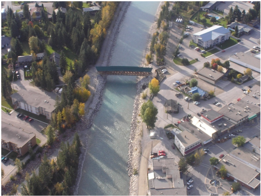
Figure 3: Covered Pedestrian Footbridge near 8 th Ave. S
