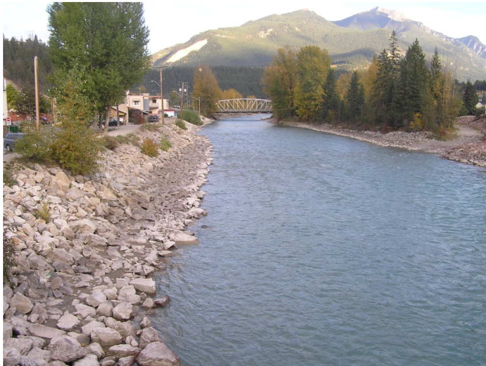
Figure 6: North Bank existing conditions
